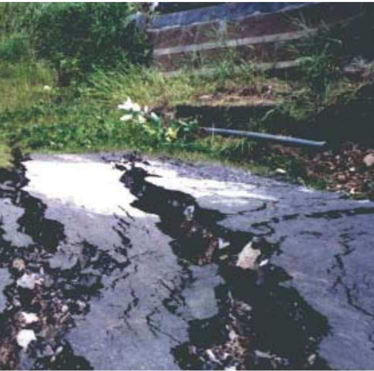
Figure 4: Ground cracking
