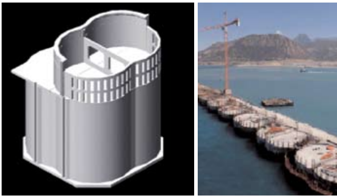
Figure 4: Detail of caisson
