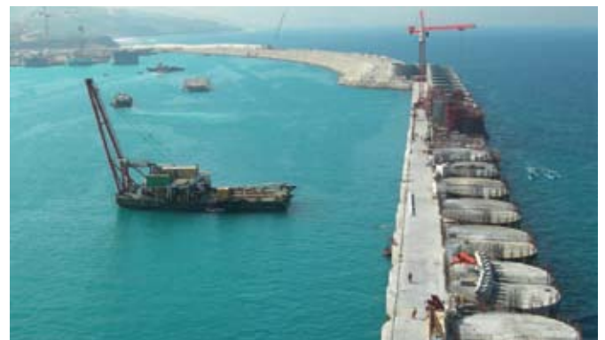
Figure 3: Detailed view of breakwater
